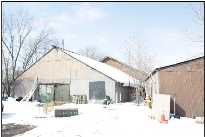
The original shop (top) is surrounded by non-historic additions on the east and north (bottom) and has been clad in corrugated-metal panels that are not original.
